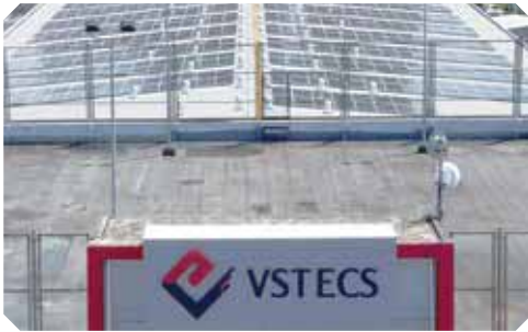
Renewable Energy Project SPS installation on the warehouse rooftop
